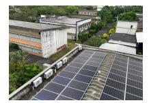
17,000 solar panels were installed on 55 buildings at the UFES main campus, Vitória, Brazil. They generate 7.7 million kWh/year of electricity, representing 45.5% reduction in the campus' electricity consumption.
