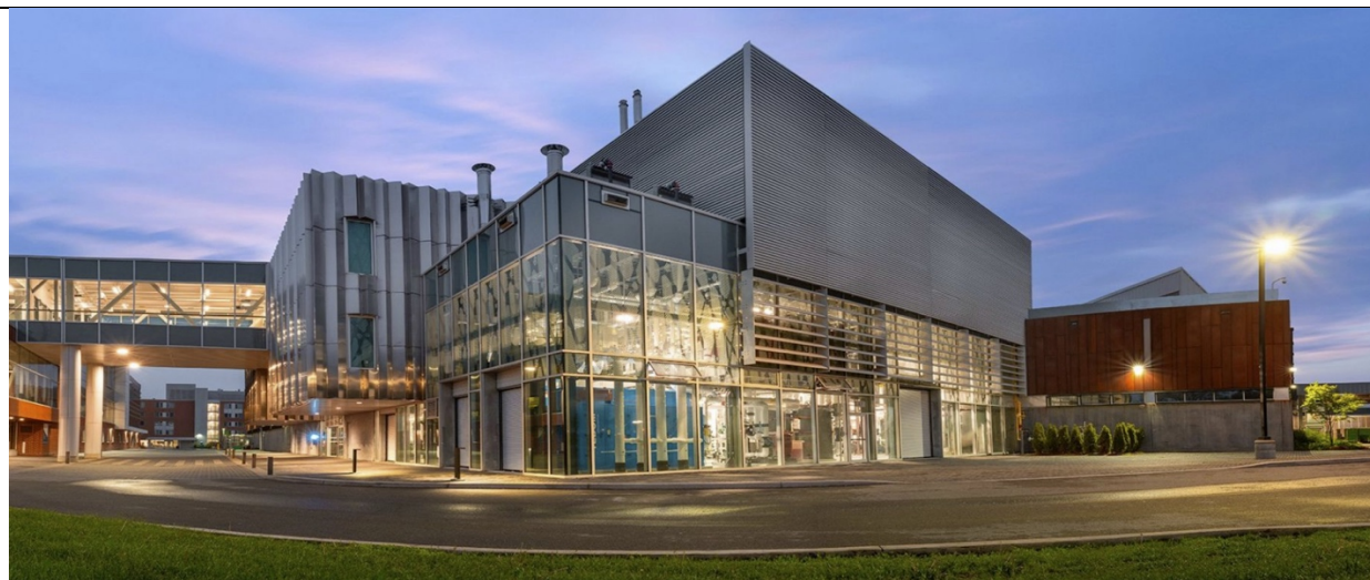
The Davis District Energy Centre which supplies heating and cooling for the campus using a combination of energy-efficient technology including combined heat and power engines and absorption chillers.
