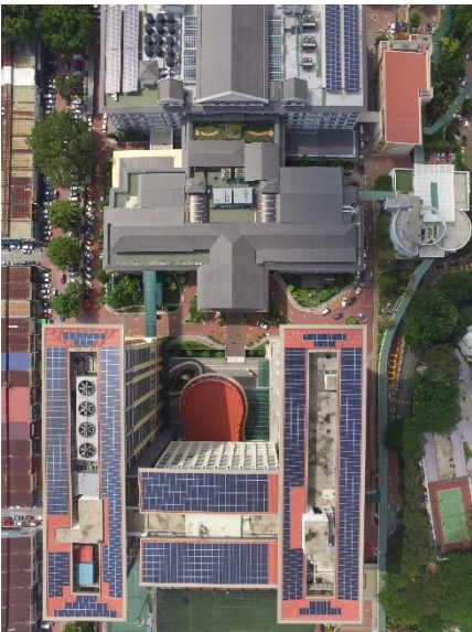
Solar Panels on Sunway University Building Roofs
