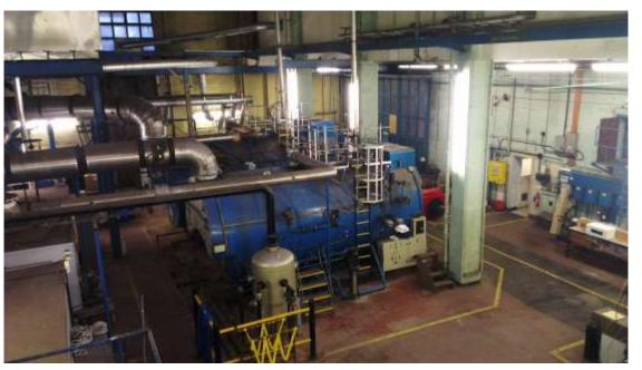
Existing steam boilers The 2No LP Steam Boilers located in John St Boilerhouse provide steam for heating and hot water to the Island Site, i.e. Royal College Building, James Weir Building, and a portion of the Thomas Graham Building now over 45 years old and at the end of their useful life
