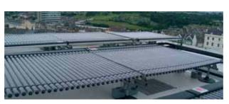
litre stainless steel pre-heat unvented cylinder and the other components of the solar heating package. The 21m  $\,^2$  of SOLARflo evacuated tubes for solar collection are mounted horizontally on the flat roof of the North Core plant room, some 28 metres above the Energy Centre.
