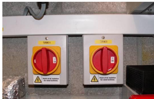
Figure 4 AC Isolators
