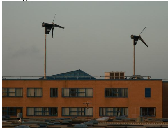
Figure 1 Wind Turbines on the Roof
