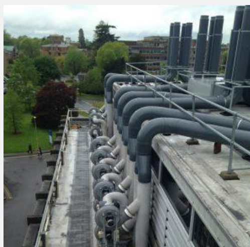
The refurbished fume cupboard extraction system. University of Reading
