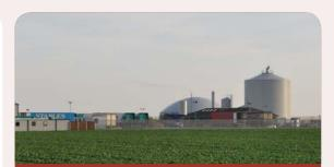
AD facilities can provide heat and power as well as replacing inorganic fertilisers. For example, this Staples facility will produce 11 million kilowatt hours of electricity every year from 40,000 tonnes of vegetable waste
