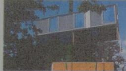
Figure 19: The solar collectors were integrated into the prefabricated modules.
