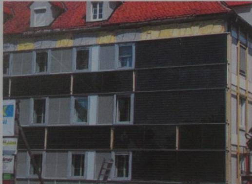
Figures 20-22: Sequence of assembly of the modules on the south-oriented facade
