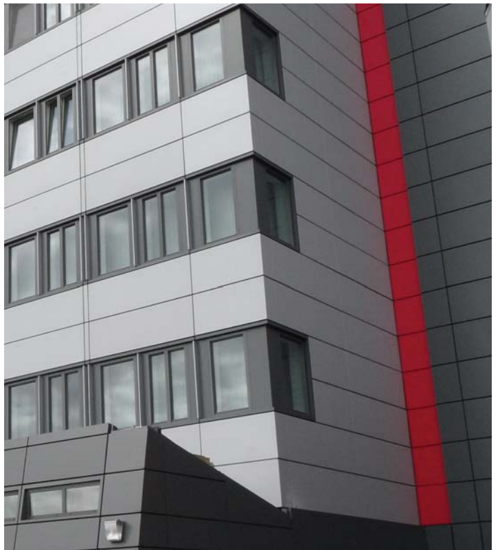
Cleveleys Building, Blackpool and The Fylde College during
