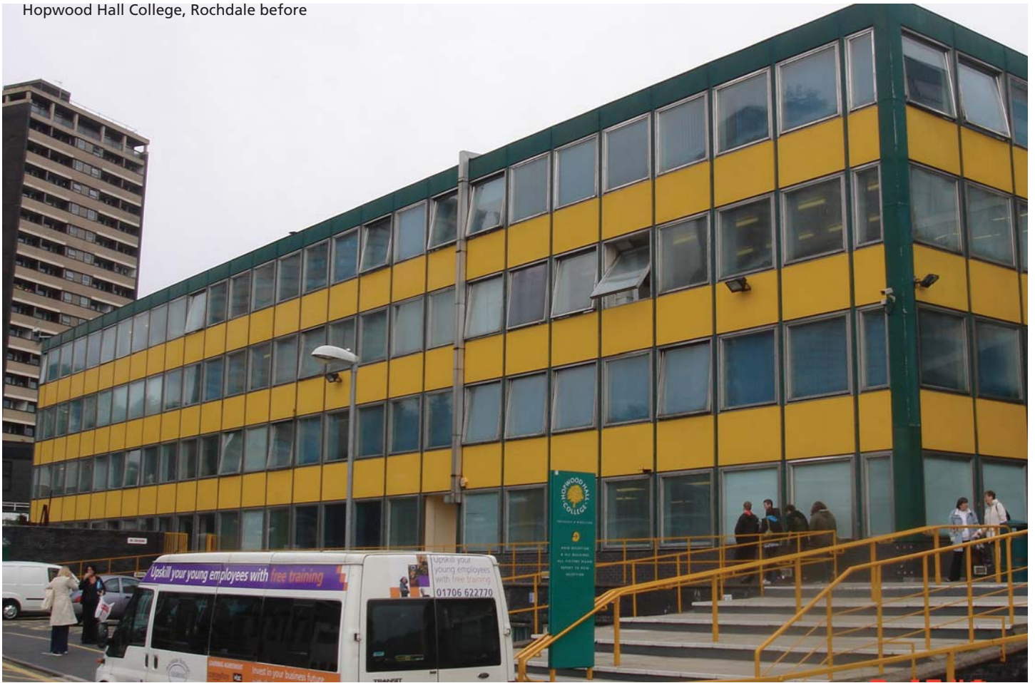
Hopwood Hall College, Rochdale before
