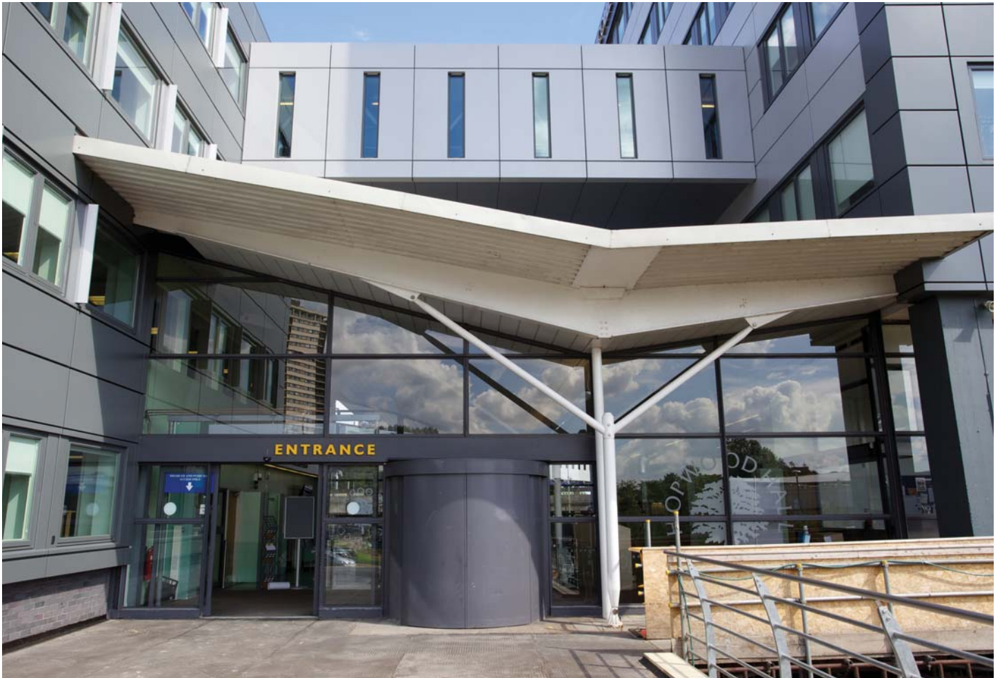
Hopwood Hall College, Rochdale after
