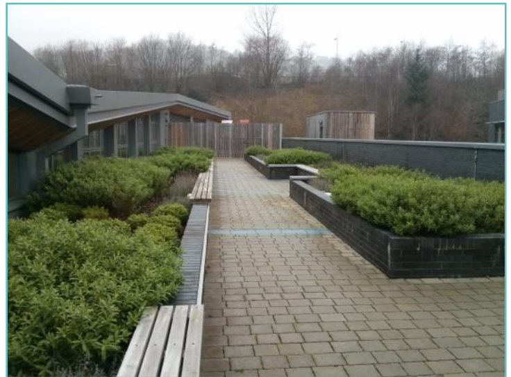
Rooftop garden: Blaenau Gwent Learning Zone
