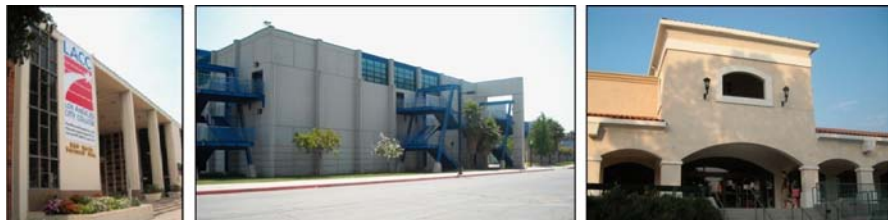
Figure 2. Los Angeles Community College District: Campus Buildings
