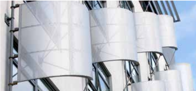
Rolle building solar shading
