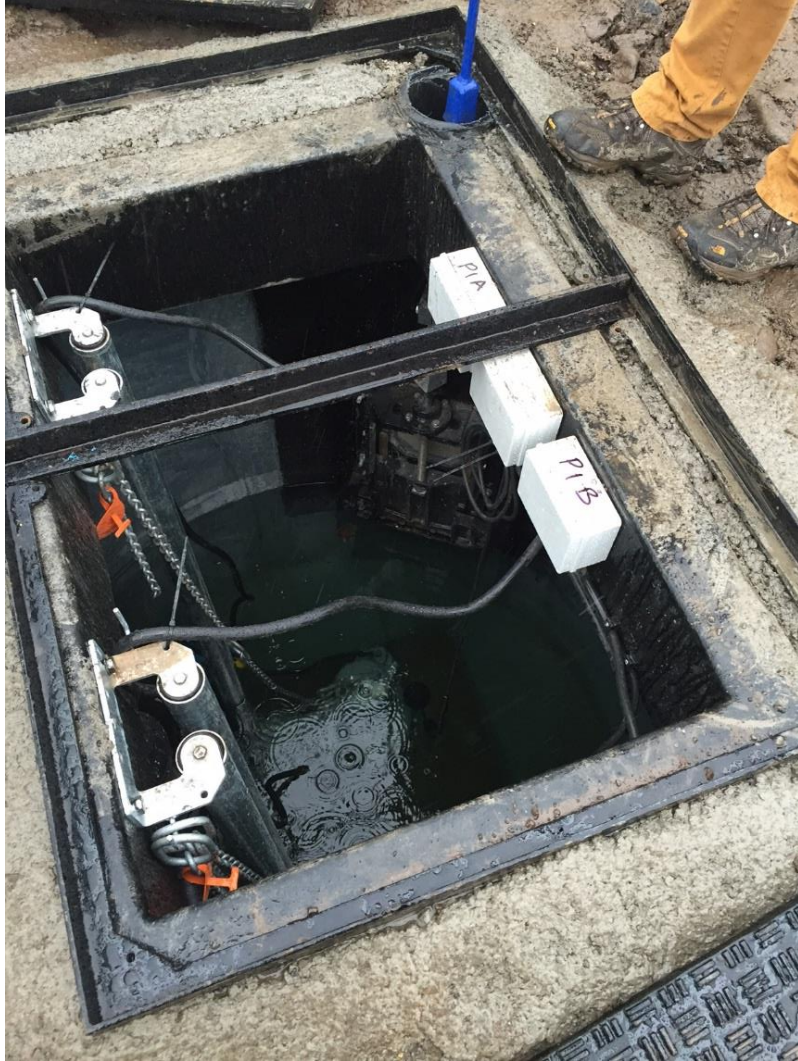
SHARC wet well incorporating a penstock into main sewer
