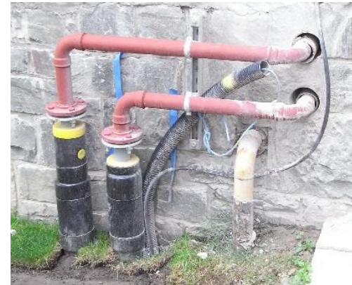
External mains into Research/labs
