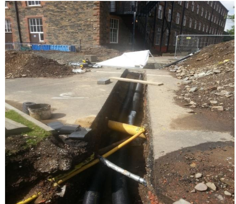
Pre-Insulated heat network external connection to High Mill
