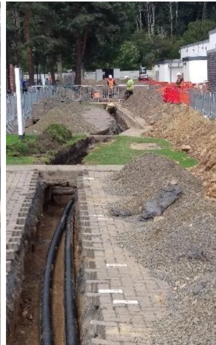
Pre-Insulated heat network external connection to High Mill
