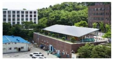
Sangji university established an on-grid, self consuming solar energy system of 50Kwp in capacity, in 2006. Since then, it has generated 128,000KWH for 30 months, saving 9,216,000KW. In the following year, the school established another solar energy system with the same capacity, generating 47,690KWH for 10 months and saving 3,433,680KW. In 2008, it installed another solar
