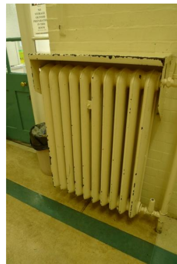
Cast iron radiators used to distribute heat throughout the school
