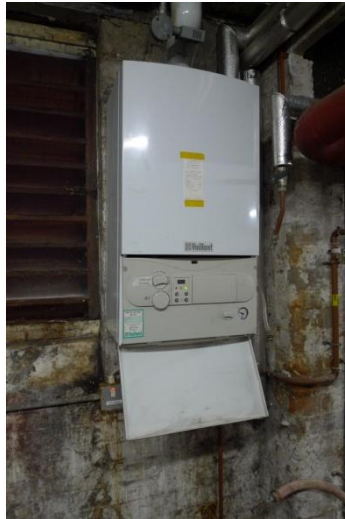
One of several standalone combi boilers used to heat areas with high energy demands
