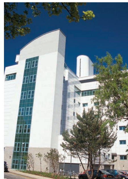
The university's second CHP system, at its King's Buildings campus, supplies heating to nearly 30 buildings including the Michael Swann Building for biological sciences. Built in 1996, the building (shown here) was named for Professor Michael Swann, under whose academic leadership the university established the first department of molecular biology in Britain.
