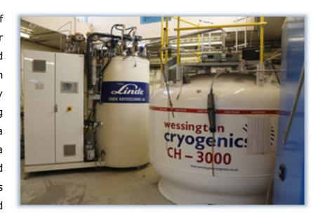
They have developed a way of recapturing the gas and returning it to the main hub, where it is re-liquefied, distributed and reused. It encompasses all existing methods/techniques of Helium recovery into one system, vastly increasing the capture of previously lost gas. This protects and futureproofs The University from dramatic fluctuations in availability and cost. At current usage rates worldwide helium reserves are estimated to be exhausted in the next 25 to 35
