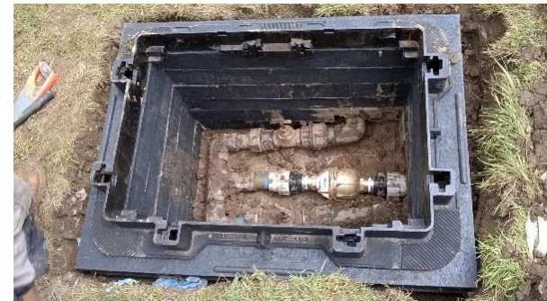
New water meter for the astroturf water cannons
